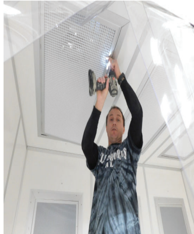
Mount covers (3) for HEPA filtration ceiling.
