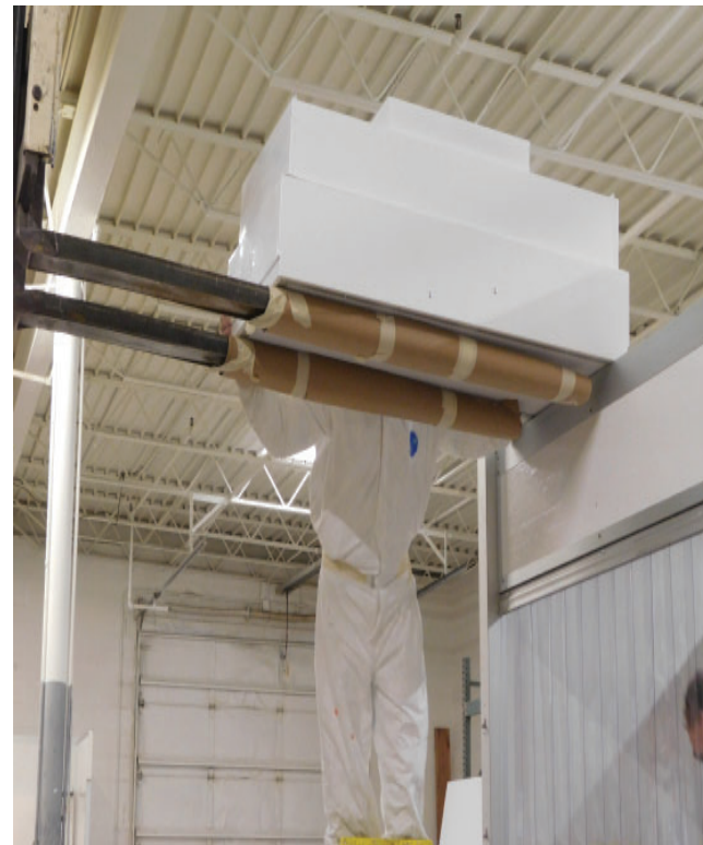
Install (HEPA Filtration unit D) using a forklift to move it into place
