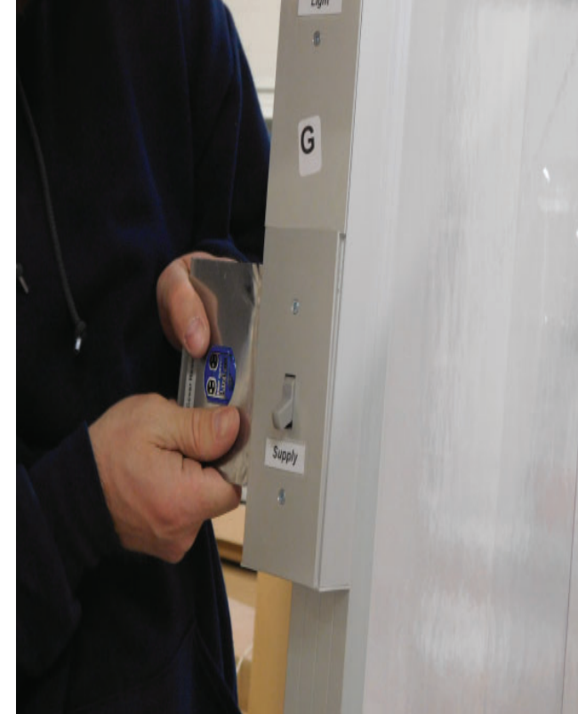
Install covers on front of (Electrical Chase G).
