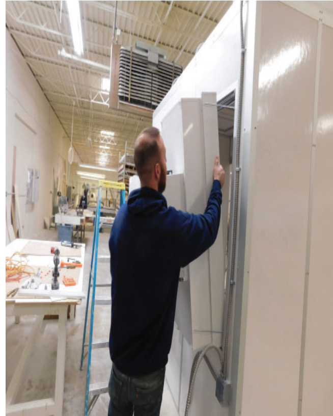
Installed (HEPA Filtration unit C).
