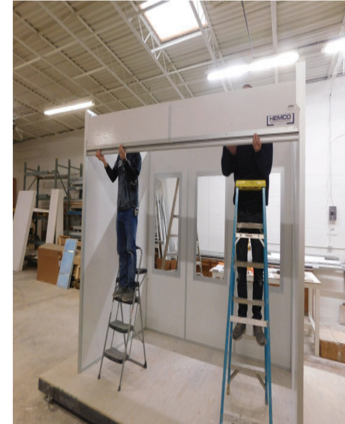
Attach (Header F) to top of Right and Left Front Walls.
