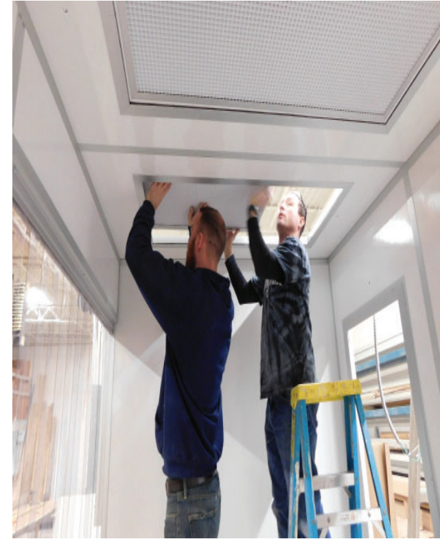
Install (HEPA Filtration unit D) into place
