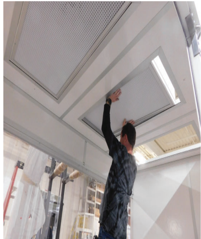
Install (HEPA Filtration unit C) into place
