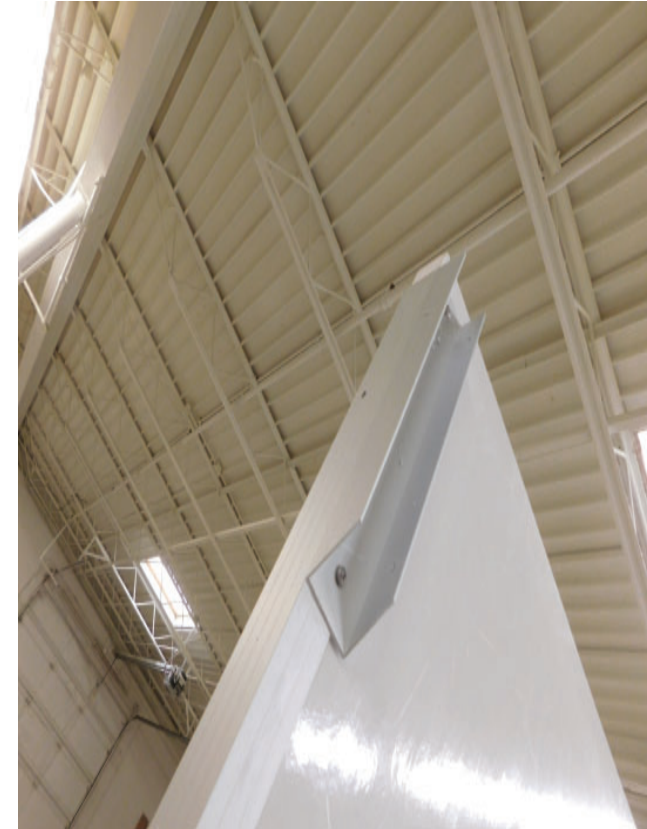
Brackets on top of Right and Left Front Walls for Headers to attach to.
