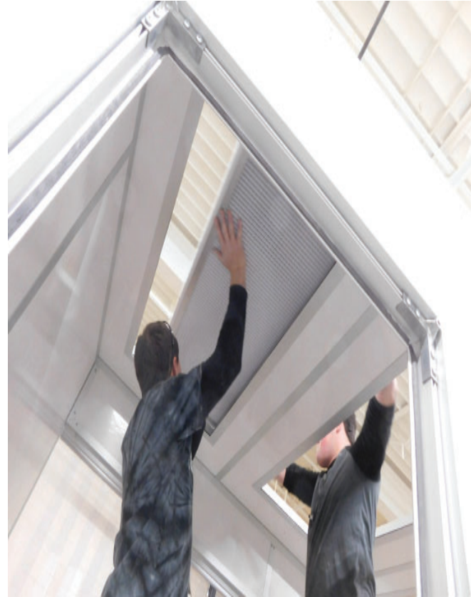
Install (HEPA Filtration unit B) into place
