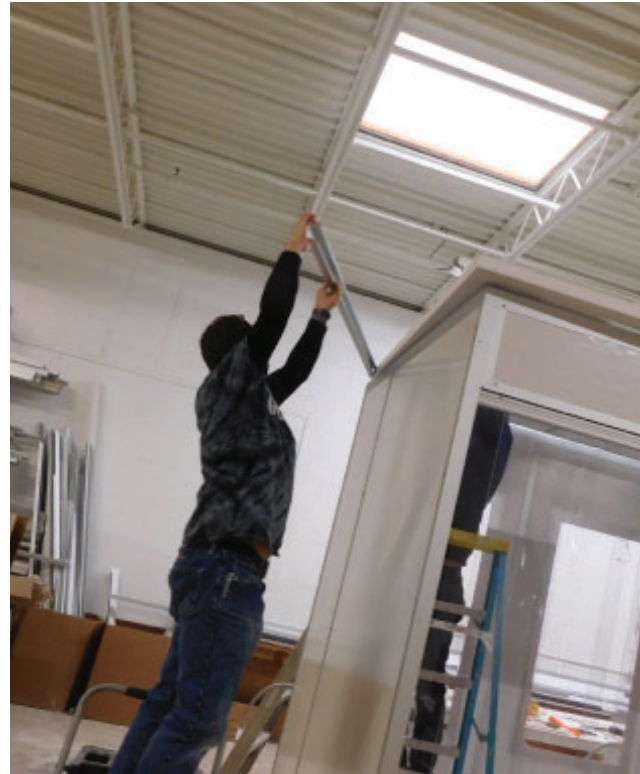
Install aluminum channels to top of Left Walls to secure Ceiling panels. Secure with provided #10 sheet metal screws.
