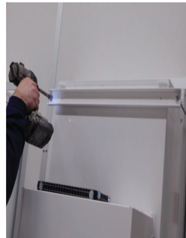
Install (HEPA Filtration unit B) attach using all thread and brackets.
