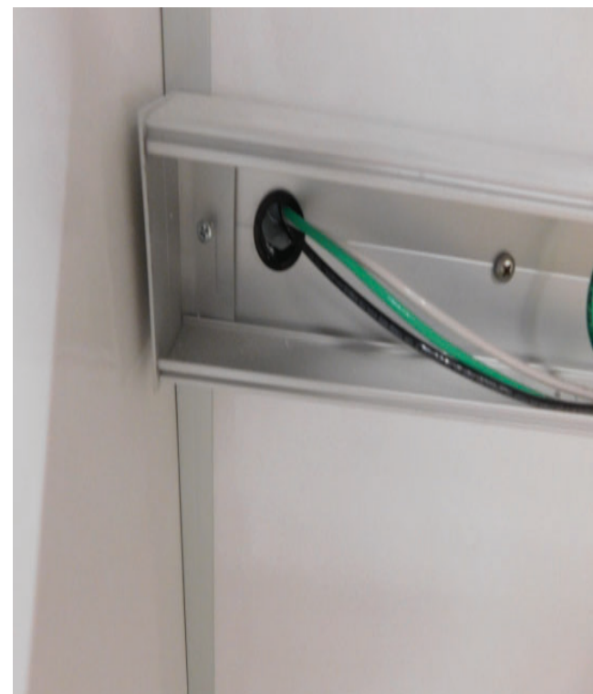
Install wires from electrical chase through back wall into electrical box on backside of wall.
